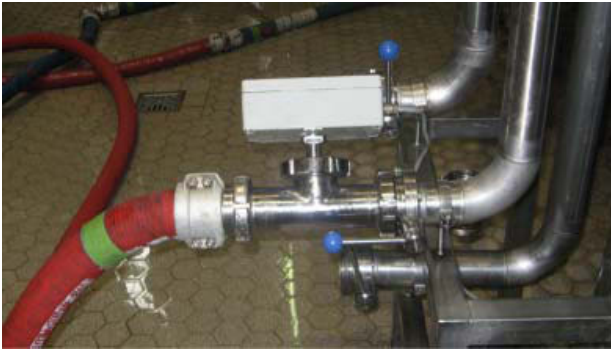
Fig. 6: STR 4115 sound velocity transmitter for interface detection at truck loading
